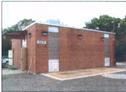
Prairie Creek Lift Station
